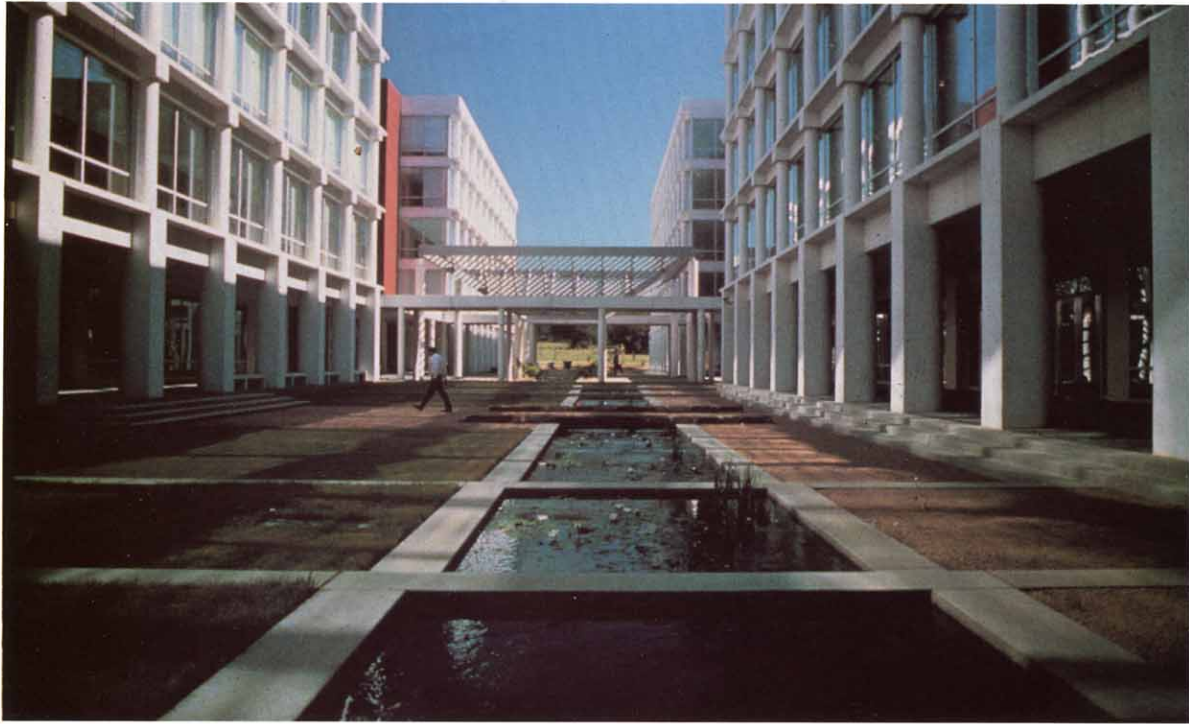
Mitchell/Giurgola Architects, IBM Westlake , detail of interior colonaded pedestrian avenue which connects the six main office buildings and features waterways and pergola-covered fountains. While the inner facing of these buildings is white precast concrete, as seen in the model below, the external facing is reddish-brown stucco.
